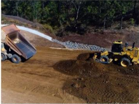
Tonka trucks are being used on the Toowoomba Second Range Crossing project. Contributed THE Toowoomba Second Range is showcasing some of road building's biggest machinery.
