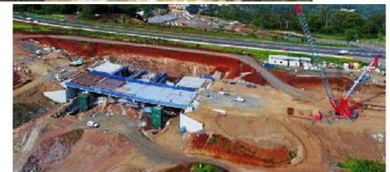
NEXUS: Works on the Toowoomba Second Range Crossing are progressing.
