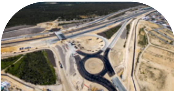
MITCHELL FREEWAY EXTENSION, WA
