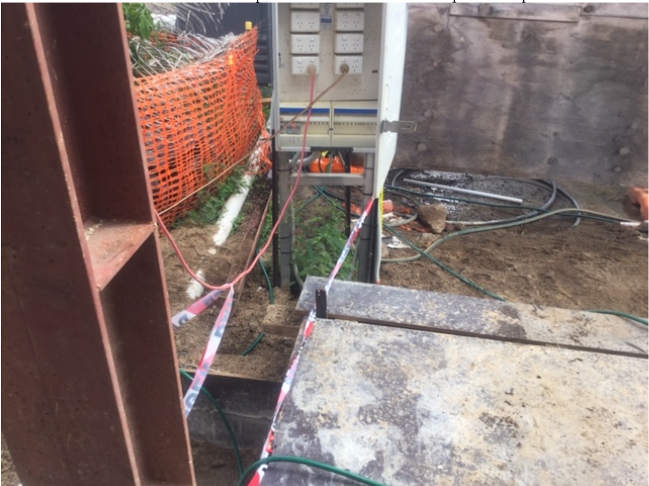
Access to a live switchboard over a drop of more than 300mm with exposed star pickets
