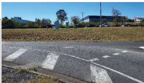
Nthbd locally traversing temp pavement
