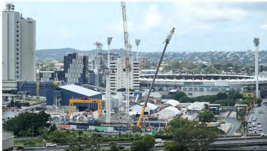
Cross River Rail's Woolloongabba Station Precinct under construction. Picture: Liam Kidston
